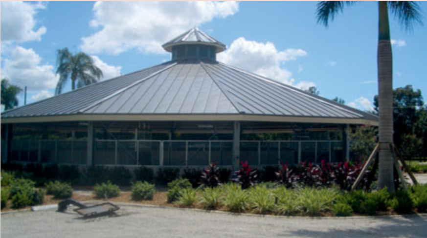
Decken-Führanlage, Double H Farm, Wellington, USA
